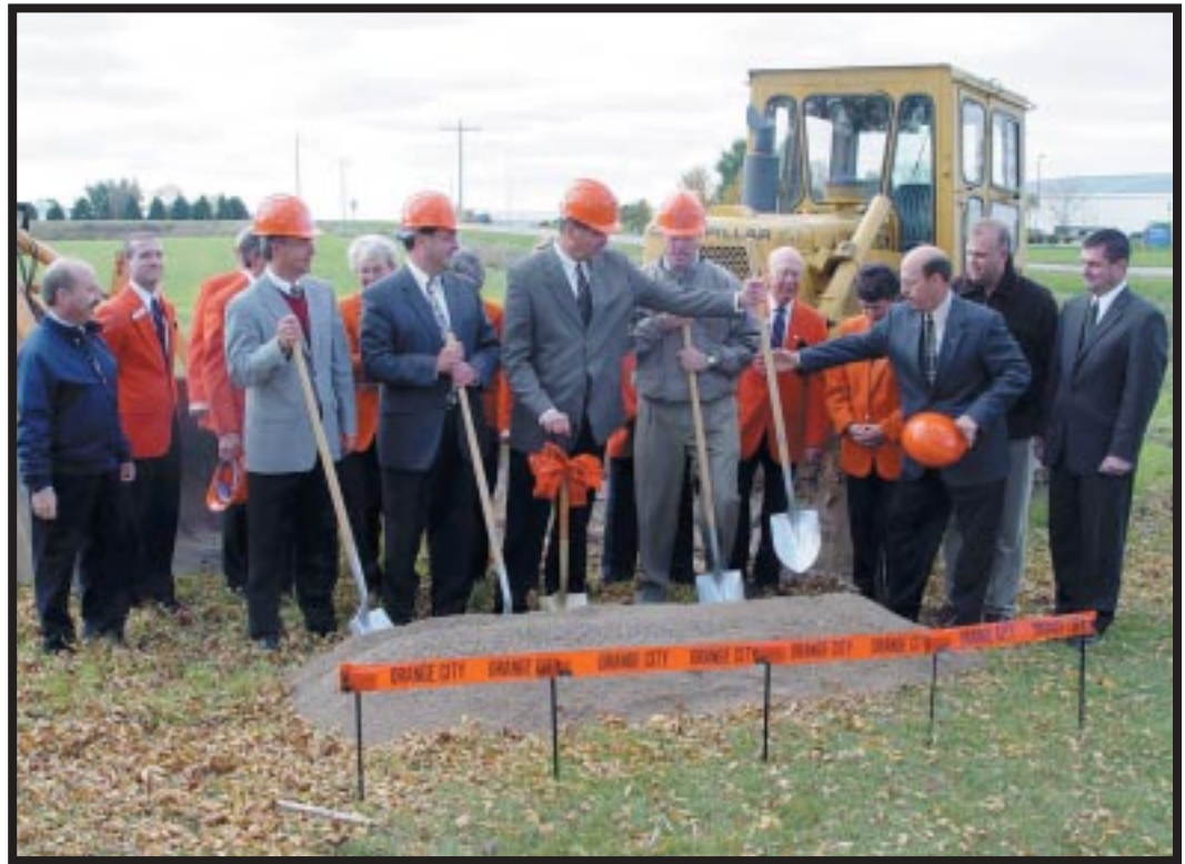
Top — North West REC participates in the groundbreaking at the new Orange City Industrial Park.
